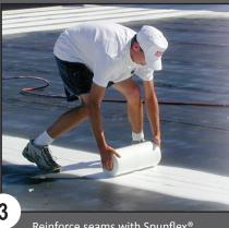
Reinforce seams with Spunflex® embedded in Rapid Roof III® Base Coat or Equinox® Base Coat.
